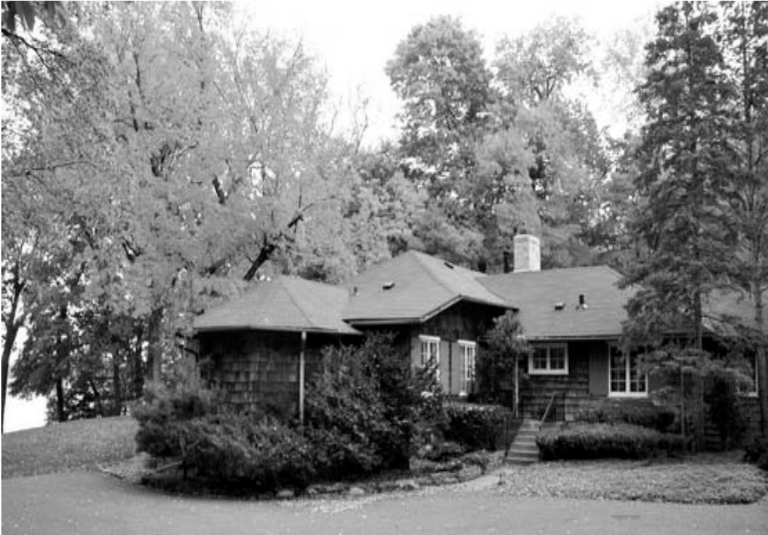
Lewis Piper House, 623 Bushaway Rd
